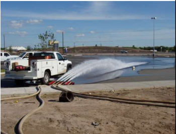
Photo courtesy of Protection Development Inc.
